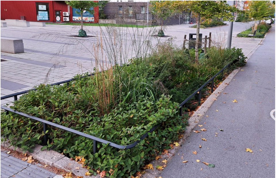
Figure 30 An "elevated robustness approach" to an urban rain garden in Rosendal, where 3-5 common shrub and grass species are planted in a relatively fine-grain pattern.
