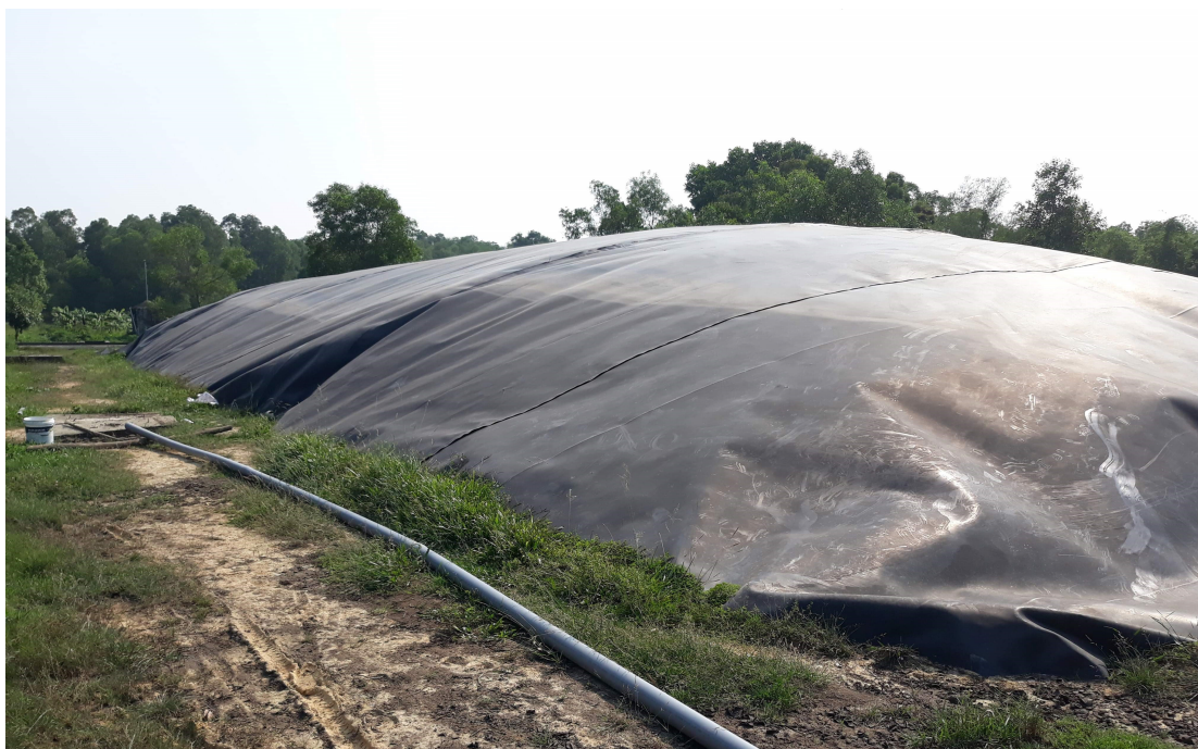
Biodigesters use manure to produce cooking gas for family home consumption. New tanks in plastic were developed that were easy and cheap to produce. In addition, the pipes and stoves were further developed.
