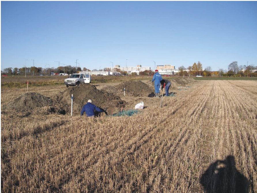
Figure 8. Excavation of dye tracing profiles during the dye tracing tests at the field sites.
